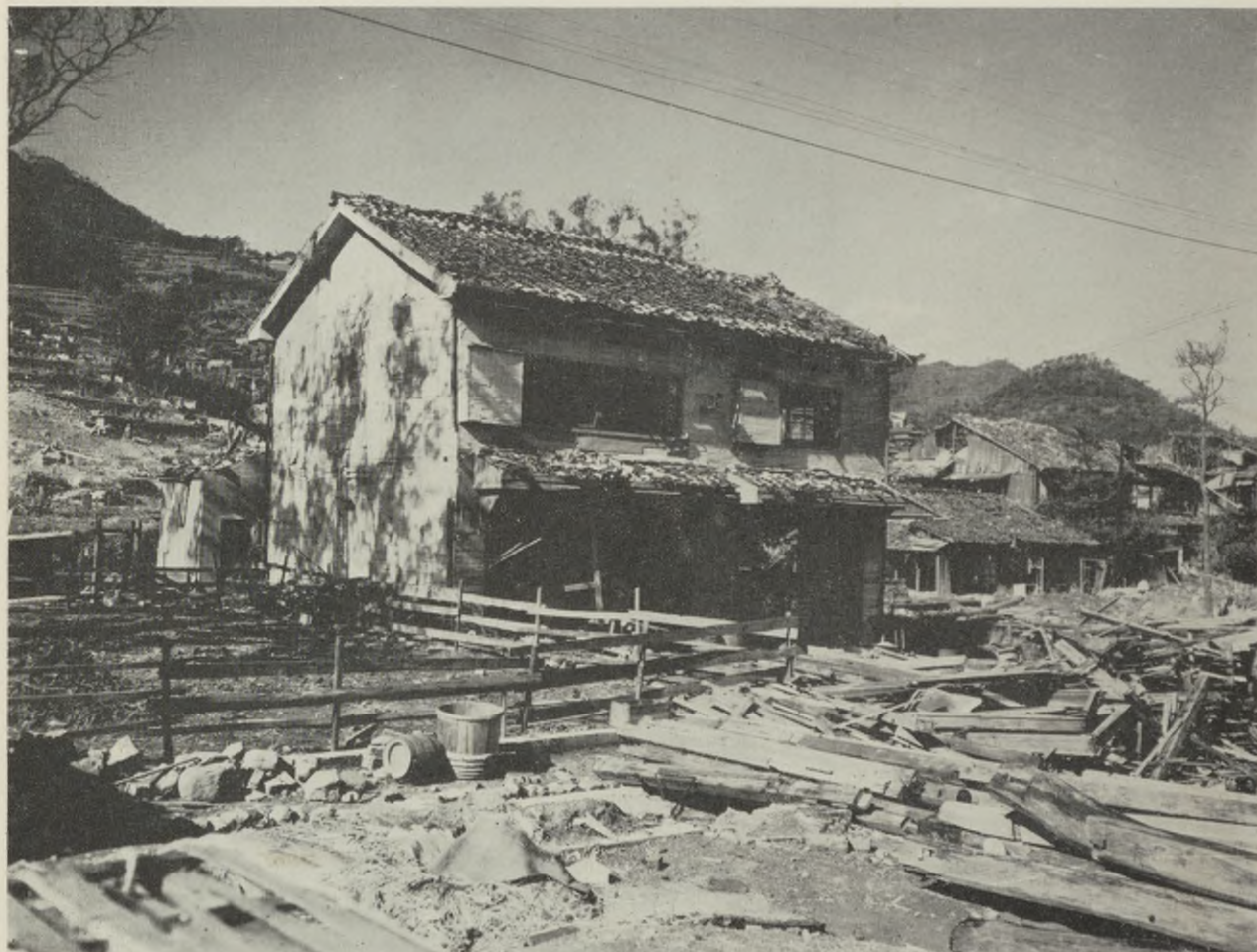
Photo 13. Inasa Substation, made untenable by a high-explosive bomb on 1 August 1945. No fire equipment or men were lost in this station.
